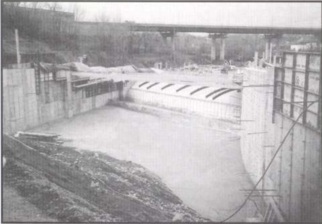
Casting ELASTIZELL EF in lifts around the Multi-Plate Arch Culvert
