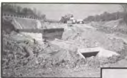
ELASTIZELL EF load balances the fill over an existing culvert to increase the grade without overloading the culvert. This eliminates the need to replace the culvert.
