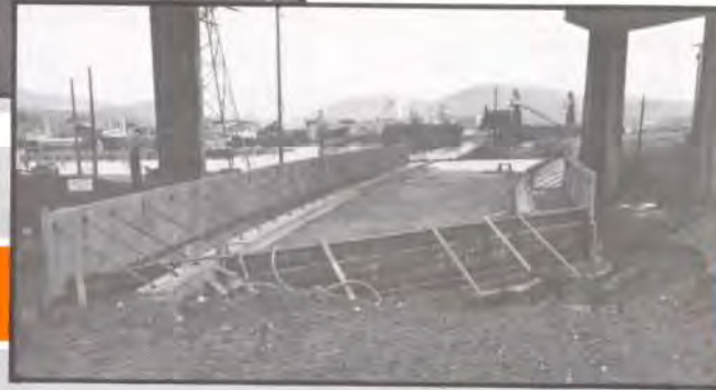
ELASTIZELL EF is placed within two rows of precast containment panels — 6' wide, 6.5' high, 4" thick.
