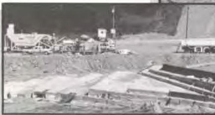
ELASTIZELL EF is engineered for load balancing to fit the sloping culvert, the depth of fill over the culvert, and the final ramp elevations.
