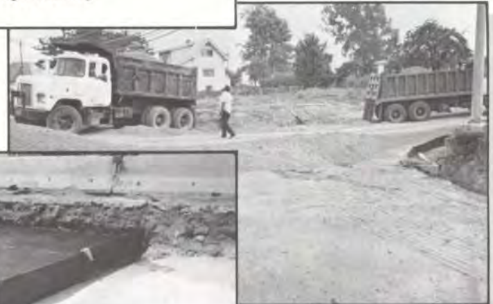
Aggregate base spread on an intersection cast with 2 feet of ELASTIZELL EF .
