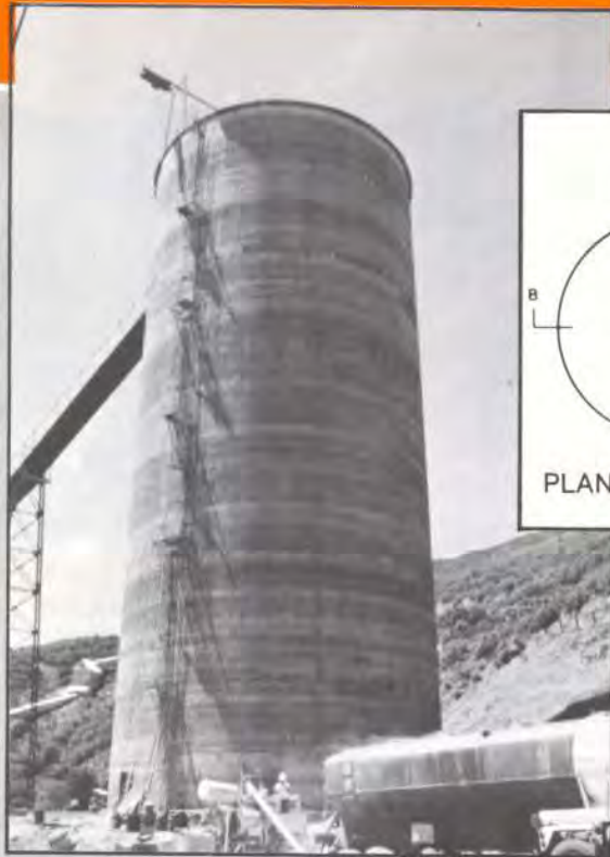
ELASTIZELL EF fills the void behind the sloping discharge hopper plates (supported by bar joists) and the slipformed silo wall.
