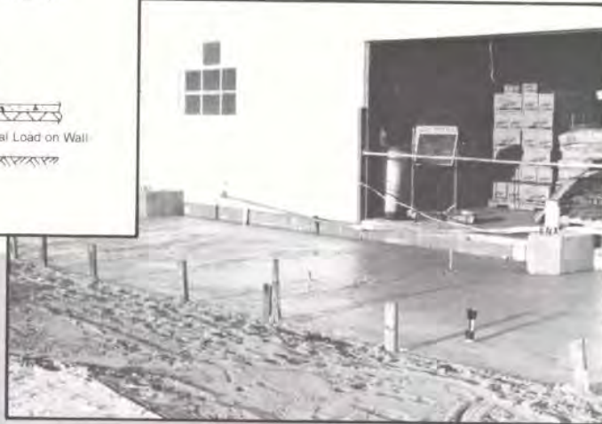
Final lift of ELASTIZELL EF ready for the finish floor slab.
