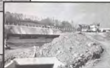
ELASTIZELL EF load balances the fill over an existing culvert to increase the grade without overloading the culvert. This eliminates the need to replace the culvert.
