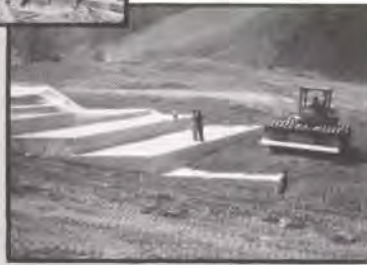
ELASTIZELL EF is engineered for load balancing to fit the sloping culvert, the depth of fill over the culvert, and the final ramp elevations.
