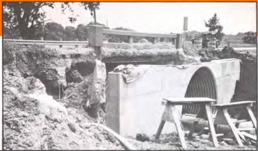
Placing ELASTIZELL EF around culvert end wall structure completely filling the void under the old bridge.
