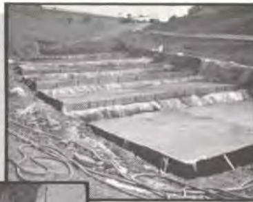
ELASTIZELL EF is engineered for load balancing to fit the sloping culvert, the depth of fill over the culvert, and the final ramp elevations.
