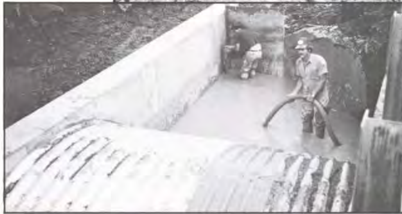
Placing ELASTIZELL EF around culvert end wall structure completely filling the void under the old bridge.
