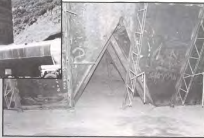
ELASTIZELL EF fills the void behind the sloping discharge hopper plates (supported by bar joists) and the slipformed silo wall.
