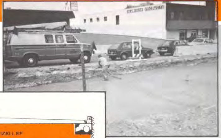
Aggregate base spread on an intersection cast with 2 feet of ELASTIZELL EF .
