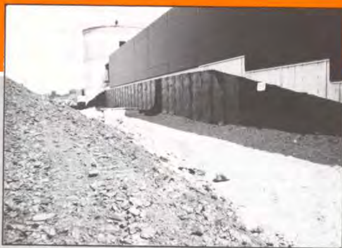
This illustrates a location where ELASTIZELL EF could be placed against the existing building wall to reduce the bending moment in the wall and create an insulating berm next to the building.
