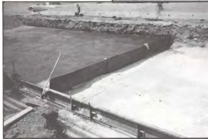
Edge forming for the second 1 foot lift of ELASTIZELL EF .
