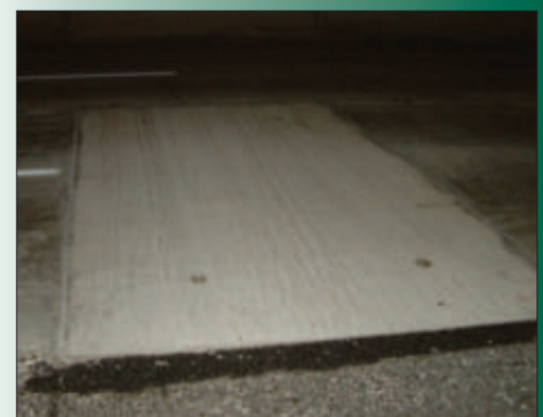
A completed concrete pavement slab repair.
