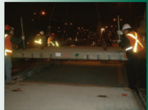
Placement of a concrete pavement slab.
