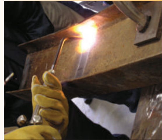
The application of a heating pattern to a steel member.
