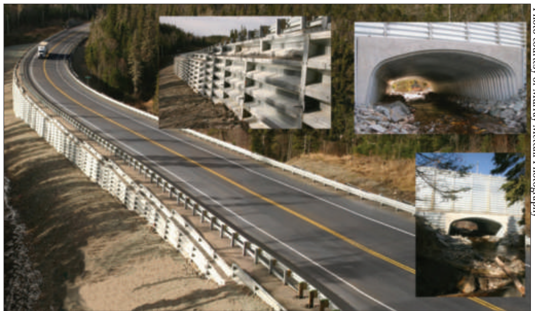
The completed roadway following culvert replacement. Top left: The steel cellular wall facing of the matrix system. Top right and bottom: The open footing structure of the completed culvert.
