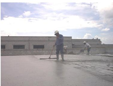
An Elastizell Roof Deck (cast-in-place), provides a slope-to-drain system, plus a strong, permanent roofing base.
