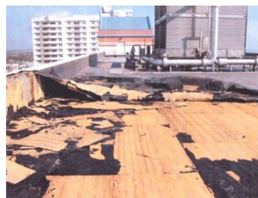
Here is a damaged rigid insulation roof deck system. All of the insulation must be replaced when re-roofing.
