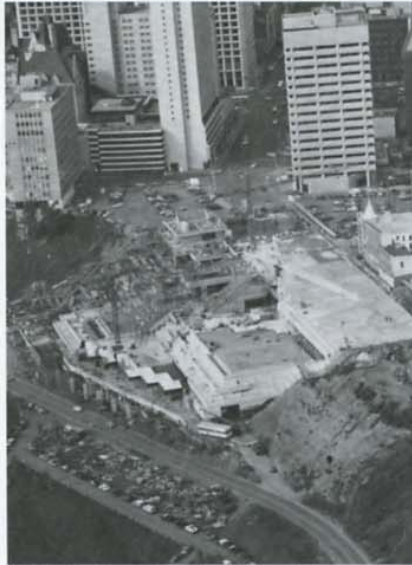
Aerial view of concrete "roof" under Jasper Avenue.
