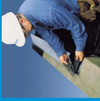
**2 Install the base flashing membrane** over primed substrate.
