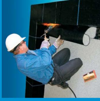
**4 Install the cap sheet** flashing membrane with torch.
