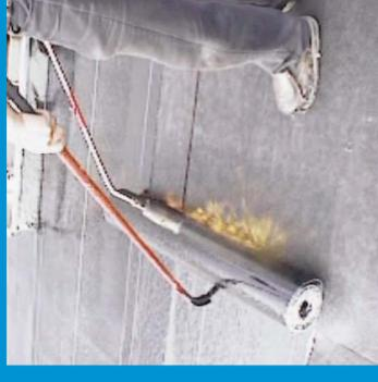
**1 Install the base sheet membrane** by heat-welding (or in a full mopping of hot bitumen or spot adhered with cold adhesive).
